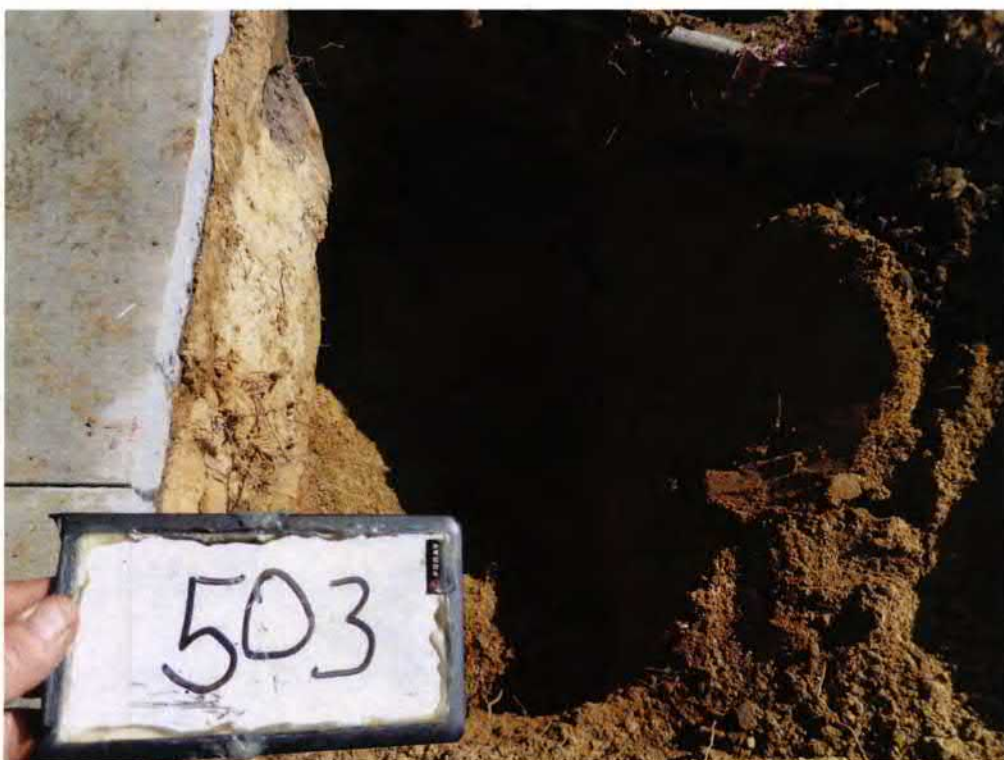
Picture 2: UST 503LaurelBB excavation.
